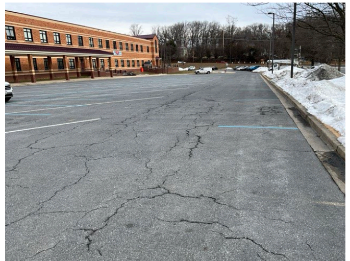
28 - SECONDARY PARKING AREA
