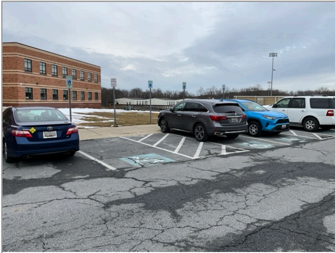
OVERVIEW OF ACCESSIBLE PARKING AREA
