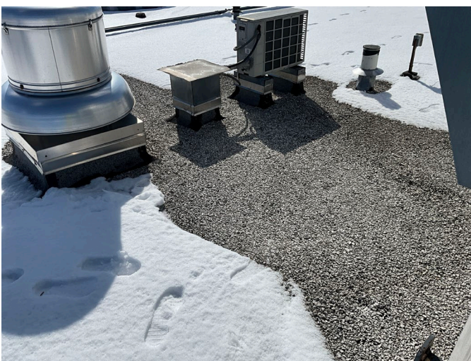
5 - PRIMARY ROOF OVERVIEW
